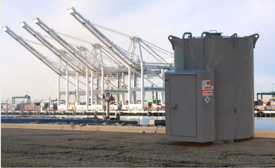
12,500 LITRE VERTICAL BULK DIESEL TANK
